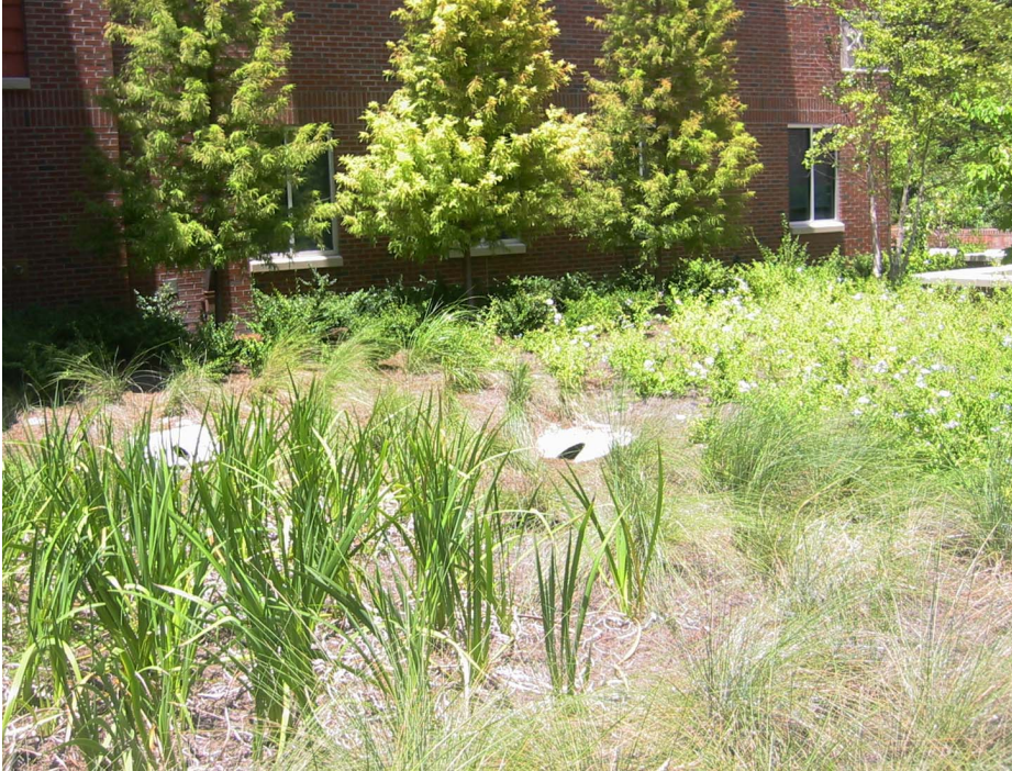
Hough Hall bio-retention stormwater treatment.
