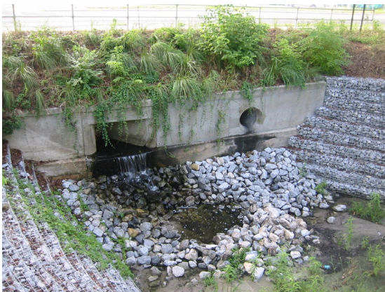
Lake Alice Creek after improvements
