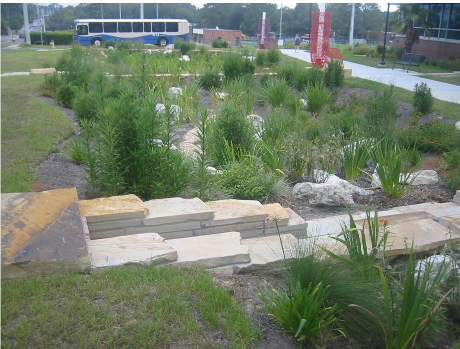
Bio-retention (rain garden) stormwater treatment at the Southwest Recreation Center.
