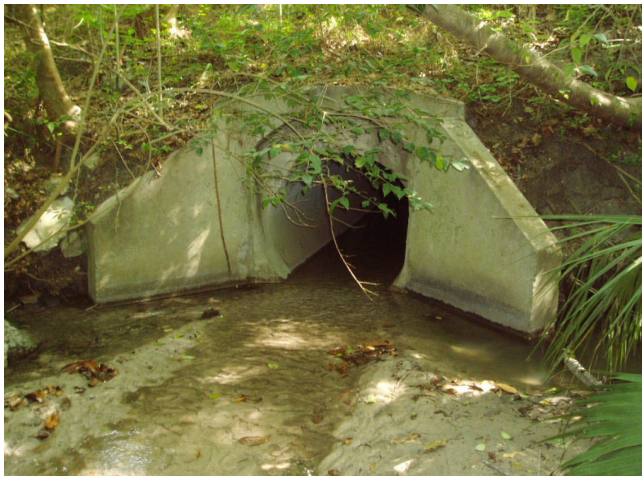
Lake Alice Creek before improvements
